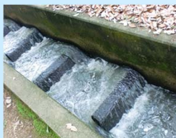
Step type in the fishway
