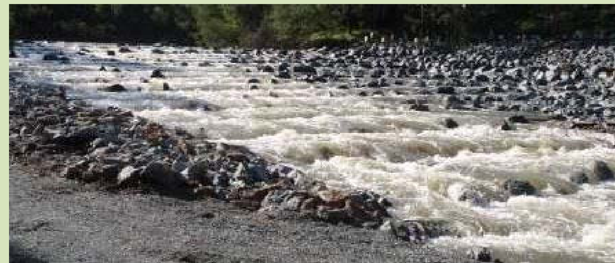
Fig.1. A typical Block Ramp Application (Rock Ramp Fishway) on Goulburn River, Victoria (© ResearchGate)
