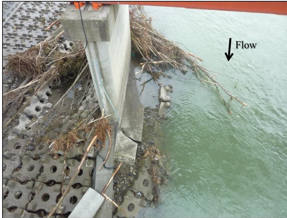
Figure 14. Damage situation of the rooting blocks (Photo taken by Okhotsk General Subprefectural Bureau Abashiri Department of Public Works Management) (Edited image of Okhotsk General Subprefectural Bureau Abashiri Department of Public Works Management)
