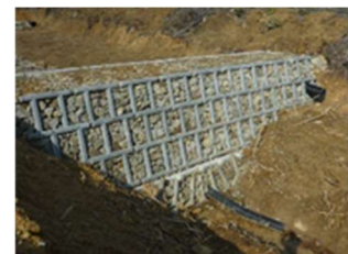
Figure 2. Example of slope construction by Ganlock method
