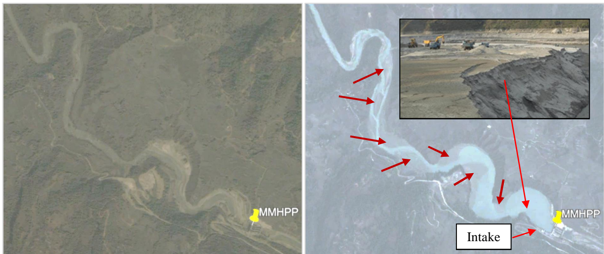
Figure 2. The reservoir of MMHPP showing narrow and almost armoured river bed before exploitation (left image) and formation of sandbars along the reservoir with severe deposition near the dam after 5 years of exploitation (right image) (Images: Google Earth)
