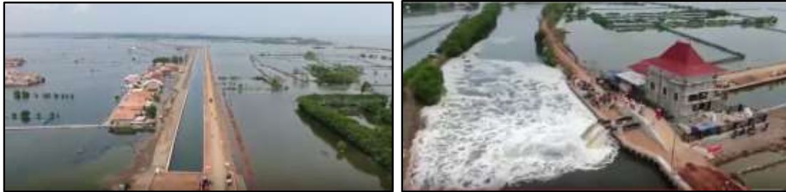
Figure 1. Sea Walls and Pump Houses in Pabean Drainage Systems
