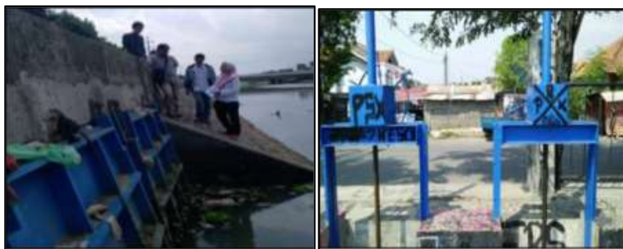
Figure 6. Type of local drainage gate inlet
