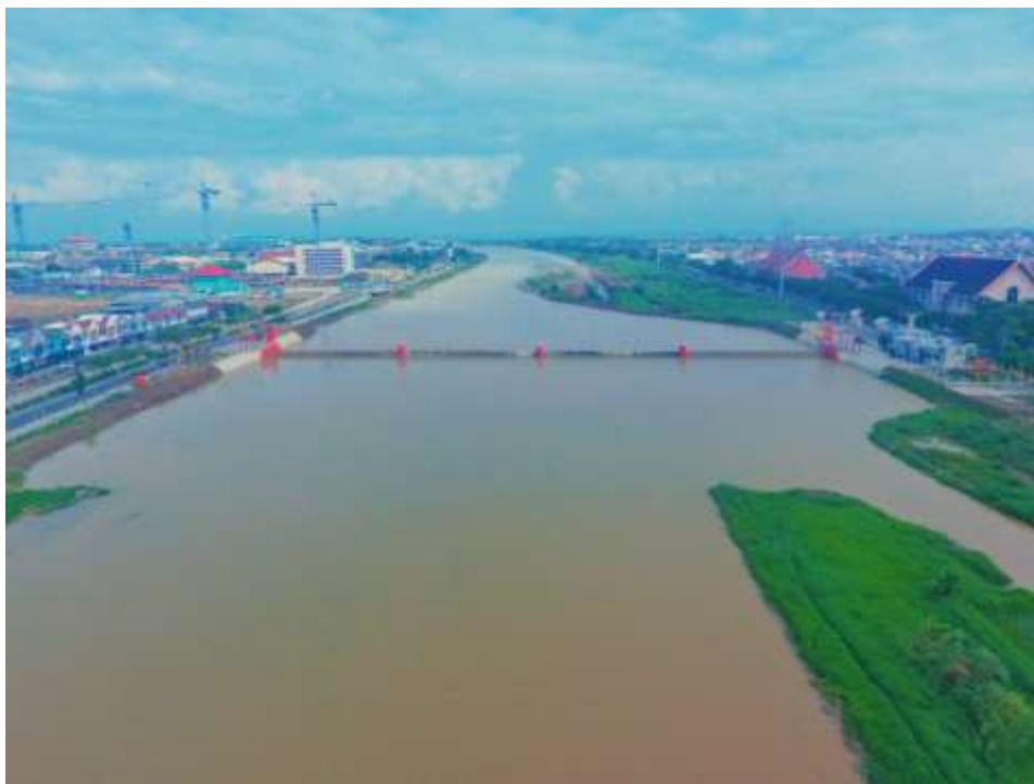
Figure 1. Location and rubber dam system downstream of the West Flood Canal
