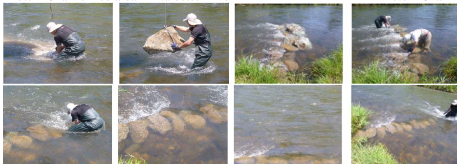
Photo 3 Installation of Stacked Boulders
