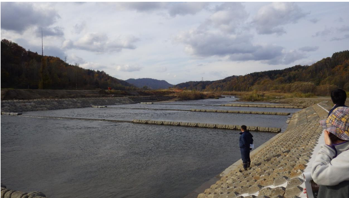
Photo 8 Installation of 19 ground sills with concrete blocks in channelized area
