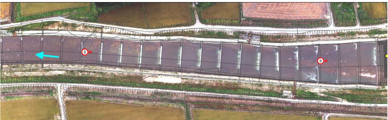
Photo 12 Gravel bed in channelized area after the installation of 19 ground sills
