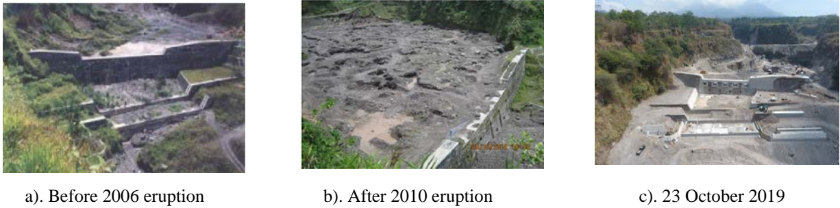
Figure 5. Topographical condition at near upstream of GE-D5
