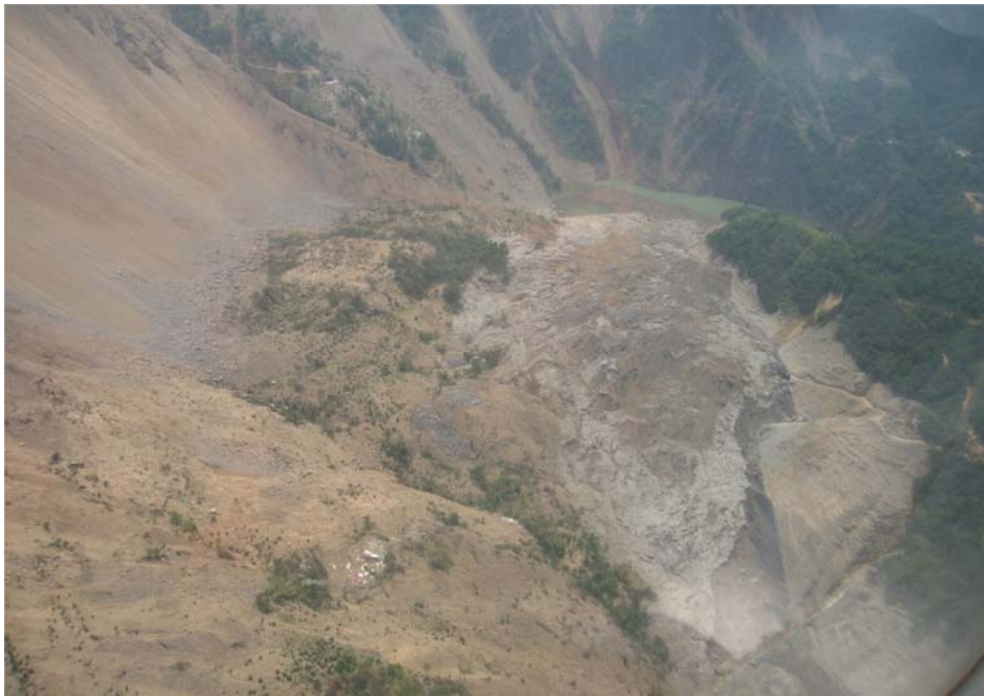
Figure 1. Aerial view of the Tangjiashan Barrier Embankment (CWRC, 2008).
