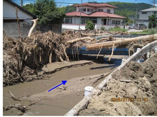
Figure 7. Sediment deposition in the downstream river channel (Downstream view at  $x'=500\text{m}$  on July 21, 2018)
