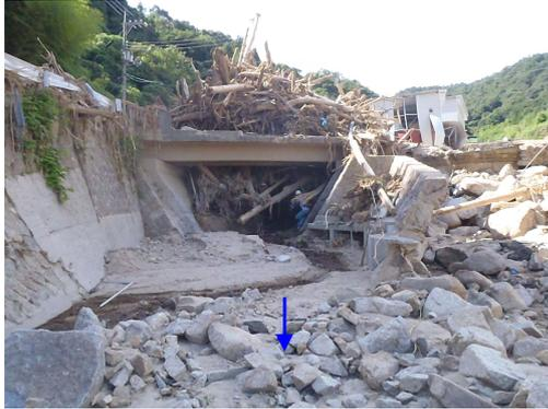
Figure 6. Driftwood trapped by Karitsudoi Bridge (Upstream view at  $x'=2,200\text{m}$  on July 22, 2018).
