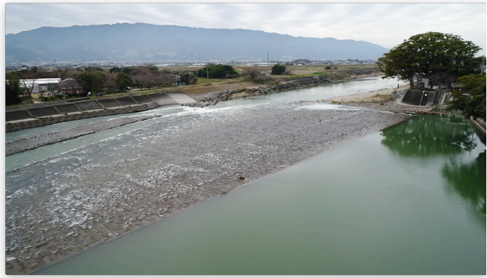
Photo3 Yamada-zeki Weir ; The intake is on the right ; the overthere is drain for sediment ; center to left is stone-paved diagonal weir ; left to overthere is main stream (Photo by Akira Ikuta with drone)
