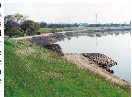
Photo.2 Stone river groynes at Kikuchi-gawa River: The darkest one was constructed by Kiyomasa KATO ; The right most groyne was constructed at 1997. ( https://www.jsce.or.jp/committee/lspd/prize/2002/works/2002b2_3.jpg )
