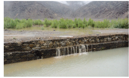
Photo10 Backing overflowed flash flood and reduces velocity by trees (Nakamura, 2017)
