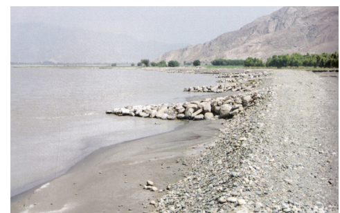
Photo11 Stone river groynes at opposite side of Mirane Weir (Nakamura, 2017)
