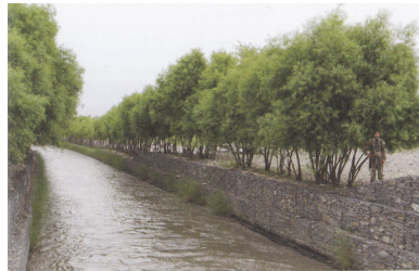
Photo9 Example of main waterway with willow trees and gabions (Nakamura, 2017)
