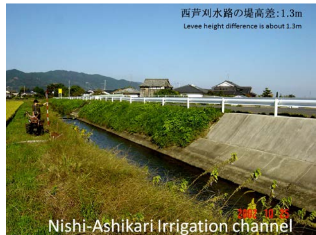
Figure 6 Nishi-Ashikari Irrigation Channel (Location and viewing direction are shown at "B" in Figure 5)
