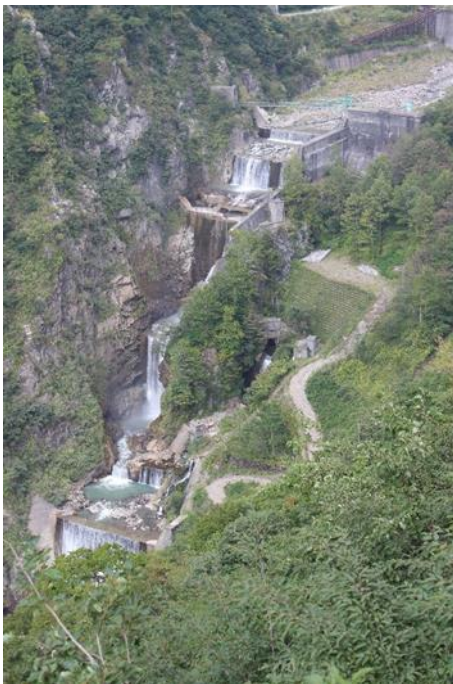
Photo 2. Shiraiwa Sabo Dam
