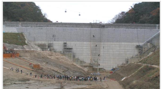
Fig. 12 Concrete Filet of Nunobiki Dam from the upstream side
