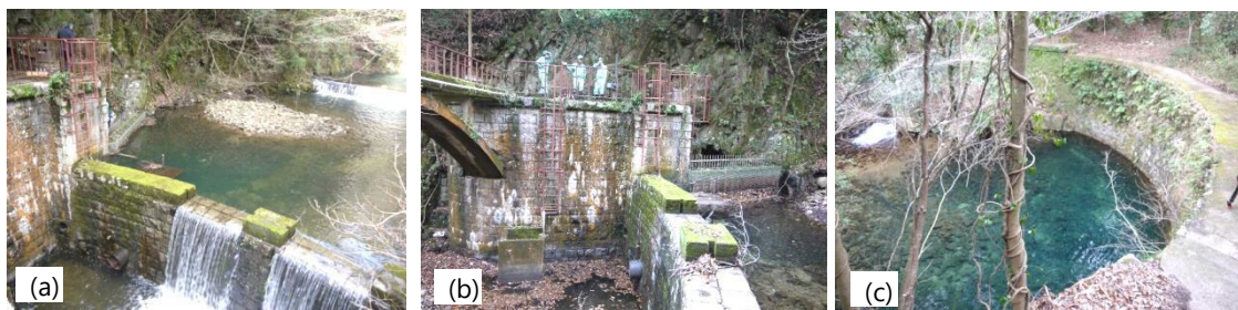
Fig. 9 Nunobiki Separation dam (a), Intake (b) and Shut-up dam(c)
