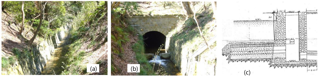
Fig. 4 Karasuhara Bypass Channel – Channel (a), Tunnel (b) and Filter to Separation dam (c)
