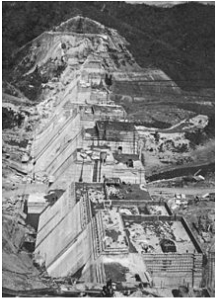
Figure 13. Katsurazawa Dam (under construction)
