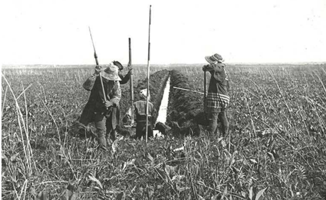
Figure 5. Channel excavation at a peatland (Tsuishikari, Hokkaido University Library)
