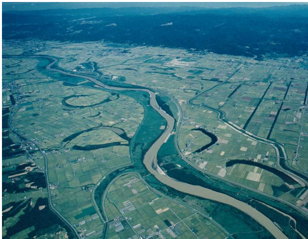
Figure 9. Cutoff works in middle reach of the Ishikari River (Hokkaido Development Bureau)
