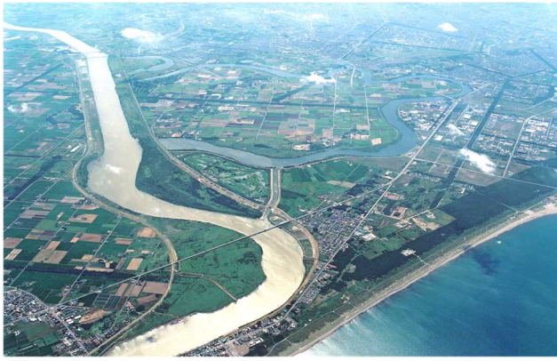
Figure 8. The Oyafuru cutoff channel
