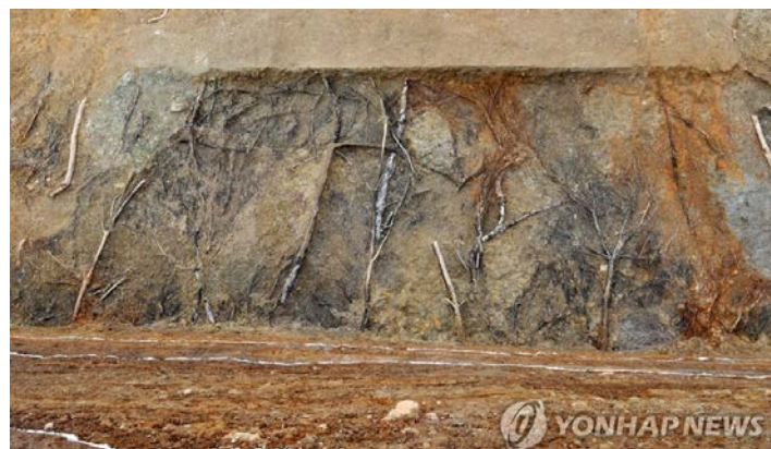
Figure 1. Yaksa-dong embankment photo taken from above (Look at the drainage-inducing technique using twigs and leaves) (provided by Yonhap news)
